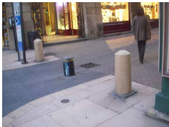
Fixed and retractable bollards controlling access to the old town.
