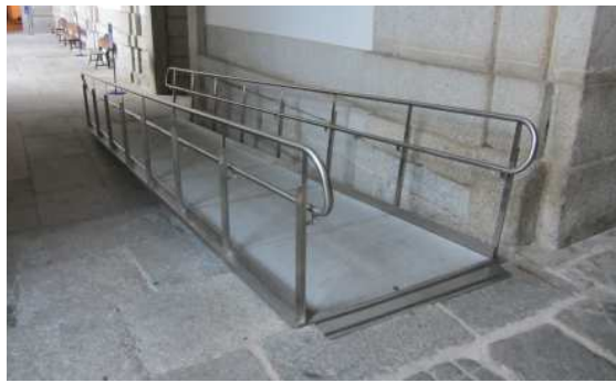
Ramp installed in Patio del Abrevadero.
