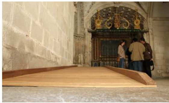
Non-slip ramp with lateral protection.
