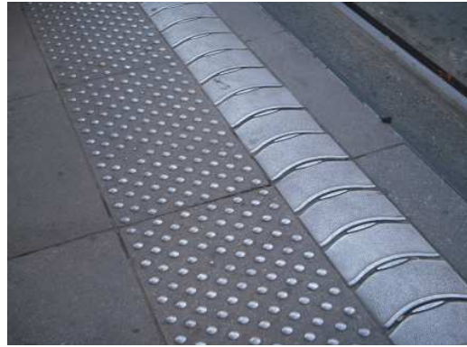
Detail of the tram stop.
