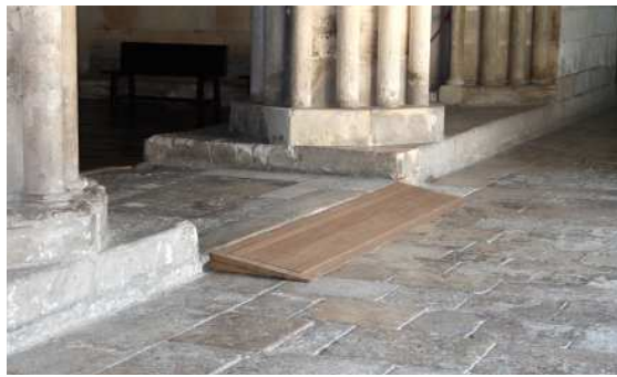
Step-ramp, made of iroko hardwood.
